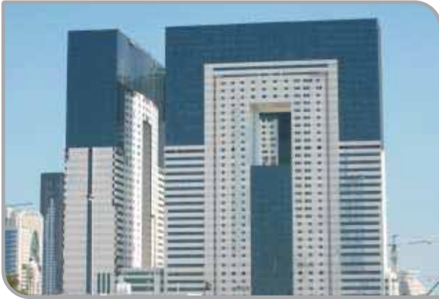
Dafna Tower 3&4, Doha
