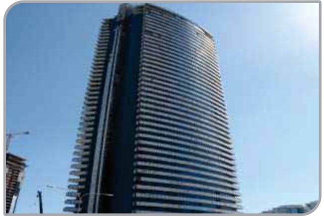
Westbay 44 Tower, Doha
