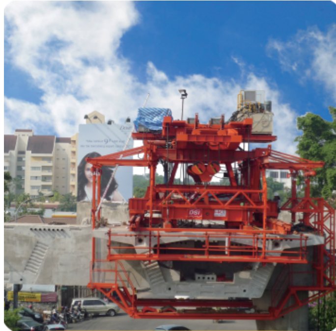
Segment Lifter with Hydraulic Winch
